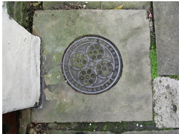
Cast iron coal hole cover, Clarendon Road
